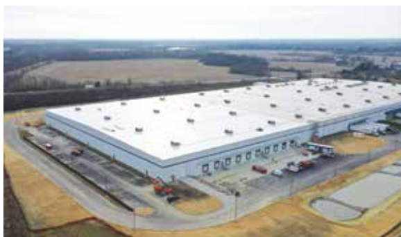
Sustainable warehouses: a high reflectivity ‘cool’ roof installation at one of Mapletree’s logistics assets in Ohio
