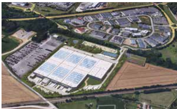
New hub: an artist's rendering of the completed Beauvais logistics facility
